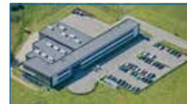
Ellab Academy Denmark
